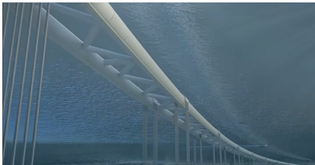
Figure 16: Rendering of a floating tube bridge proposed for crossing Sulaffjorden (a fjord) as part of Norway's E39 coastal highway project.
